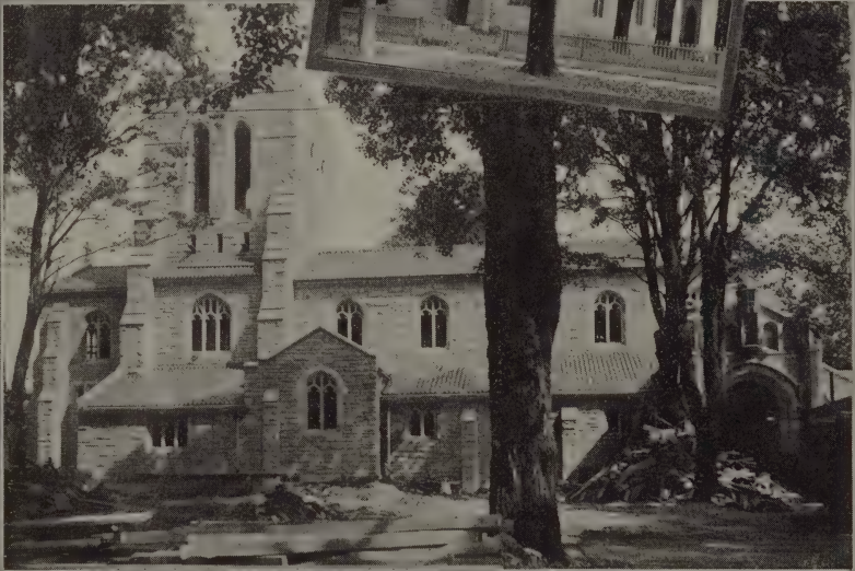
NEW EPISCOPAL CHURCH IN COURSE OF CONSTRUCTION
